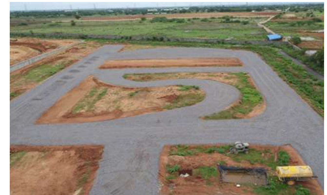
Test-tracks for Autonomous Vehicles
